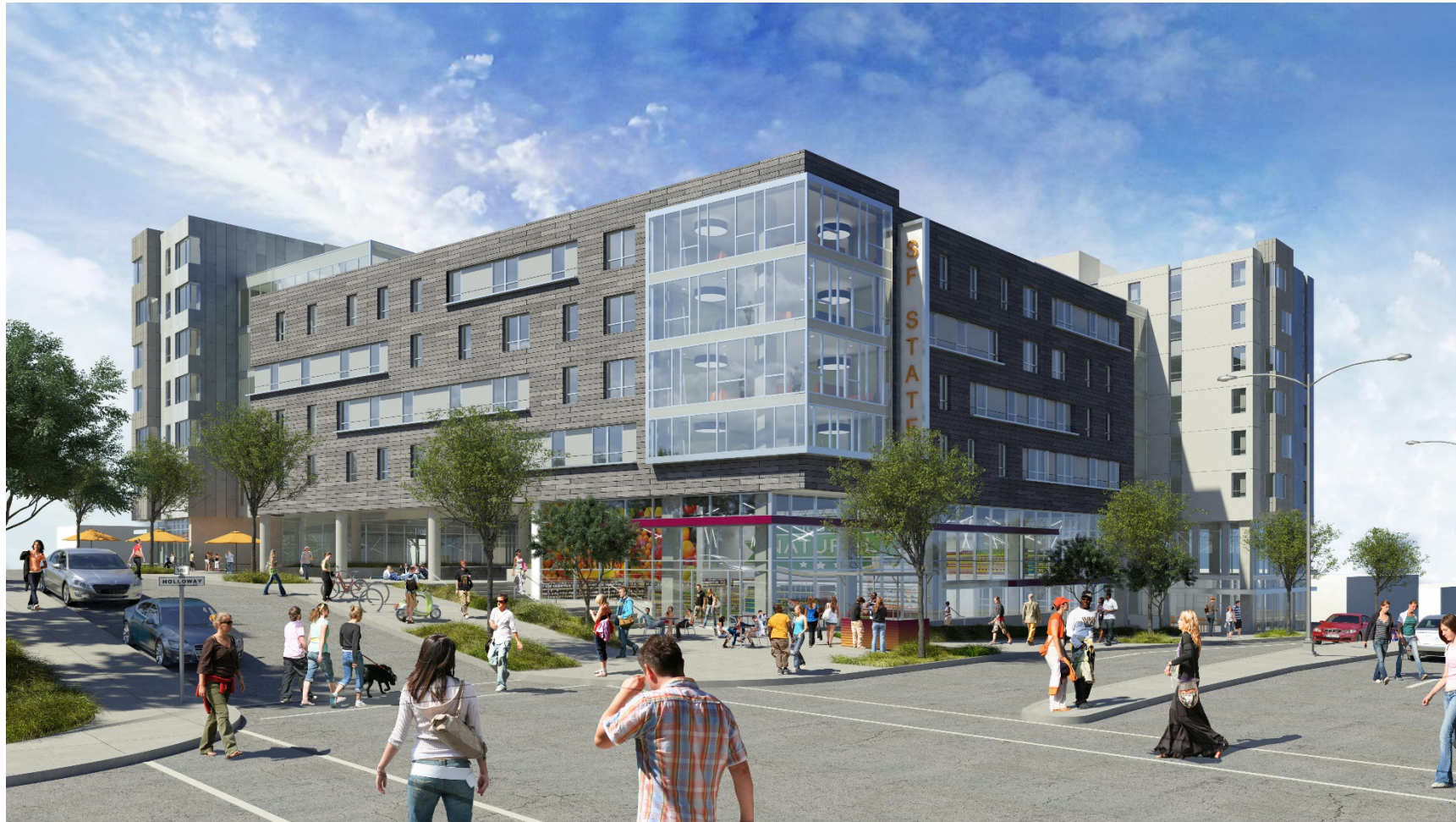
Holloway Revitalization Project
